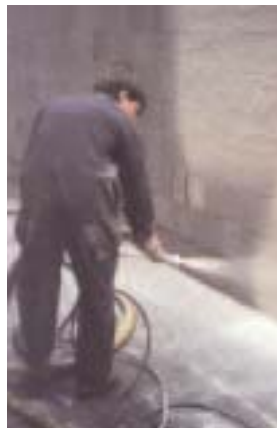
Spraying Pre-mix GRC Render
