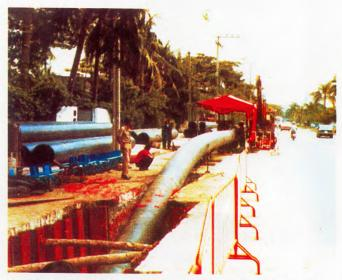
Relining of old leaking water pipeline in Bangkok, Thailand. Dimensions ø 355 - 710 mm. Total length 9 300 mm.
