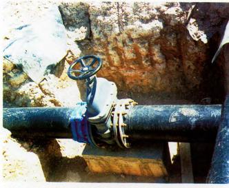
315 mm ø Sewage line connected with gate valve in Oman
