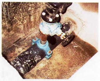
200 mm ø HDPE pipe connected with air valve in Oman
