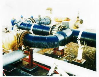
Replacement of Carbon Steel pipes with HDPE for crude oil with all interconnections, in Oman.
