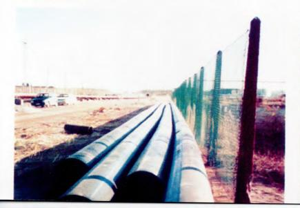
200 mm ø HDPE pipe installed above ground in rocky terrain in Oman
