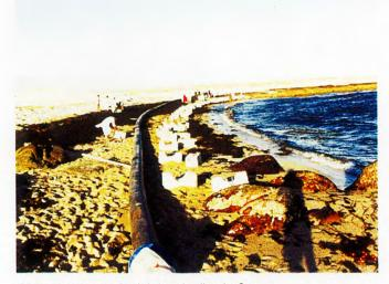
315 mm ø seawater intake pipeline in Oman.
