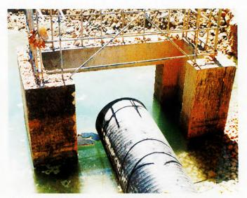
$600\ mm$  to  $1200\ mm$  ø HDPF Weholite pipes for storm water drainage at port, in Oman.
